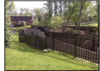
Clockwise from top: Caroline Weltzer; Margaux McGlasson; Circle Drive/Grand Ave. Storm Water Improvement Project
