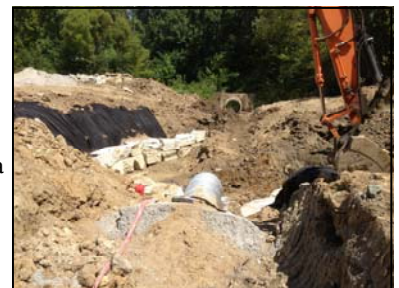
Below: Photo of Niblack Stream Restoration project
